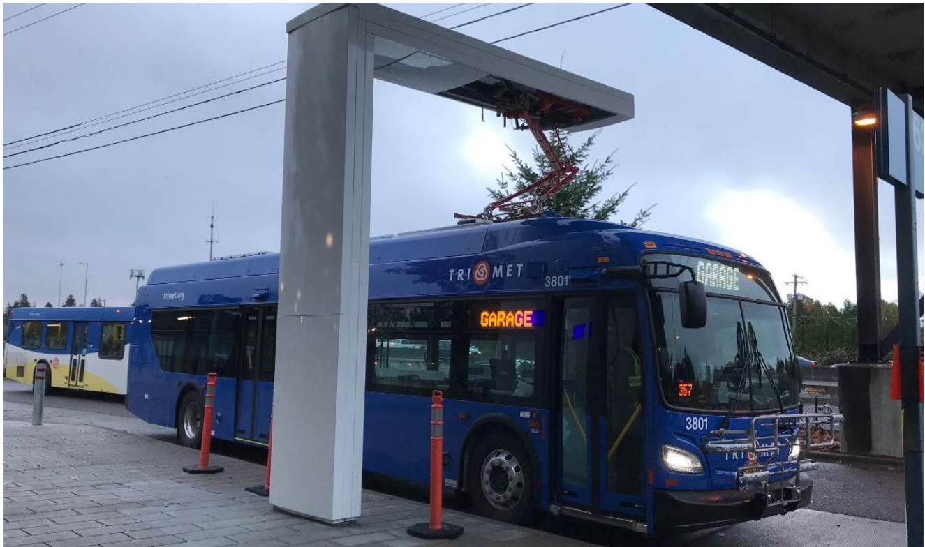
New battery electric bus now in service with overhead charger at Sunset Transit Center
