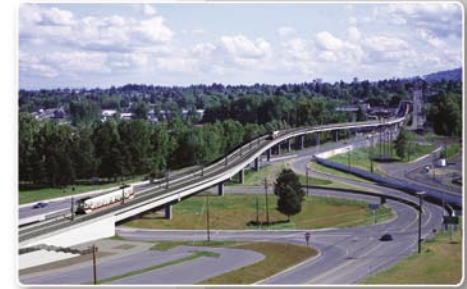
• The 1,000-foot Vanport Bridge (above), spanning the Columbia Slough.
