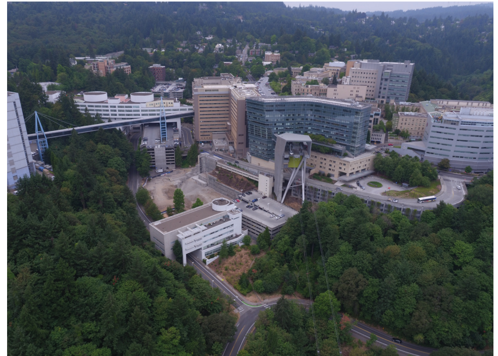
2018 aerial image with Elk's Children's Eye Clinic under construction
